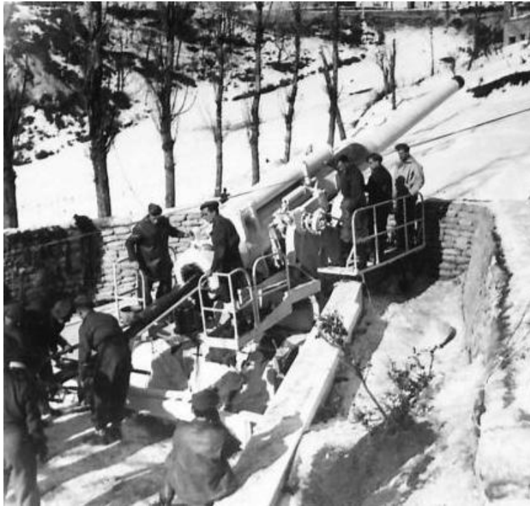
Figure 29 – The 54 th Heavy' only operational 8in Super Heavy gun, in action near Loiano, on 22 nd December 1945. The weapon appears to have been painted white to blend in with the snow covered landscape. The gunners are currently loading in a shell, using the two-man lifting cradle, which is then pushed into the breech using a long pole.
